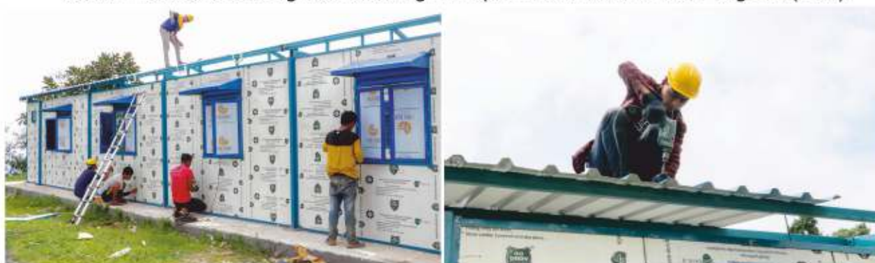
Trained candidates constructing modular hospital at Chiephobozou CHC
