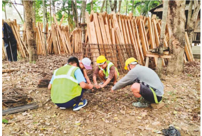
Assistant bar bender & steel fixer during their OJT training binding of stirrups in column and footing challis
