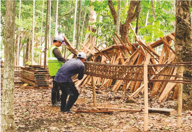
Assistant bar bender & steel fixer during their OJT training binding of stirrups in column and footing challis
